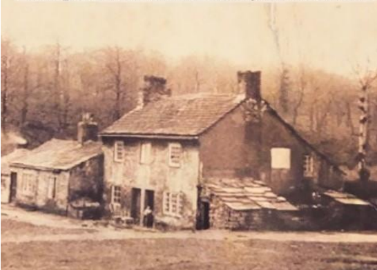
Cottages at the bottom of Dyehouse Lane
